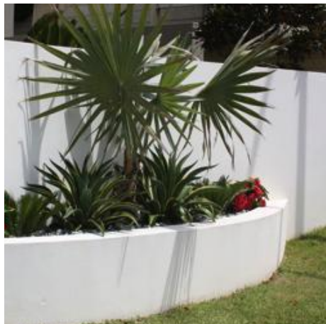
Tiered Painted Block Work Retaining Walls
